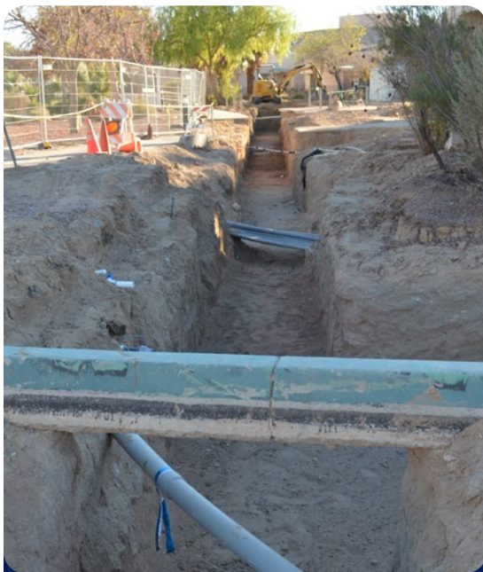
Hydronic piping repair is currently an ongoing project at the Home.
