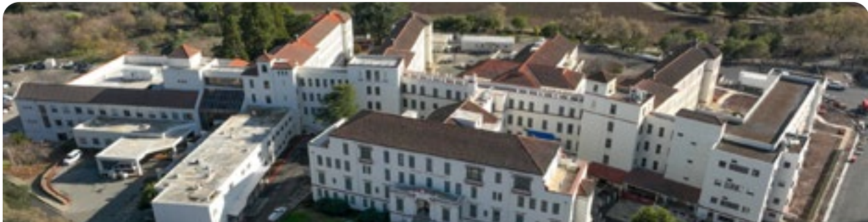
Aerial view of the Holderman Skill Nursing Facility.
