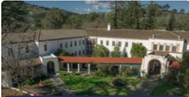
The Wilson Hall domiciliary building.
