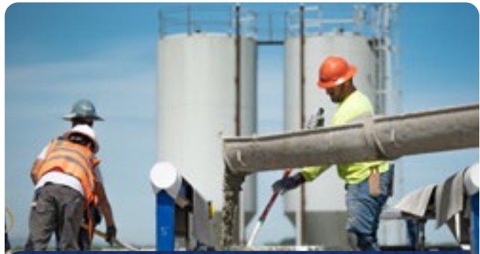
Pouring concrete for the walls of the new SNF.
