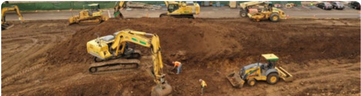
Construction work begins at the new SNF.
