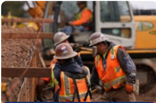
Workers building a retaining wall at the new SNF.
